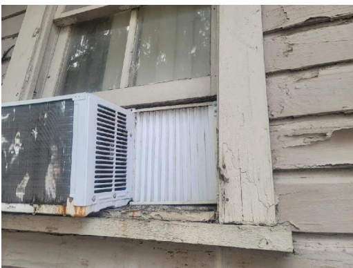
Exterior(001) D-Wall, Center Wood Window Components Lead-Positive, Deteriorated
