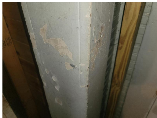
Hallway(005) A-Wall, Center Wood Door Jamb, Casing Lead-Positive, Deteriorated
